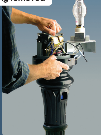
Open ballast housing with tray being removed
